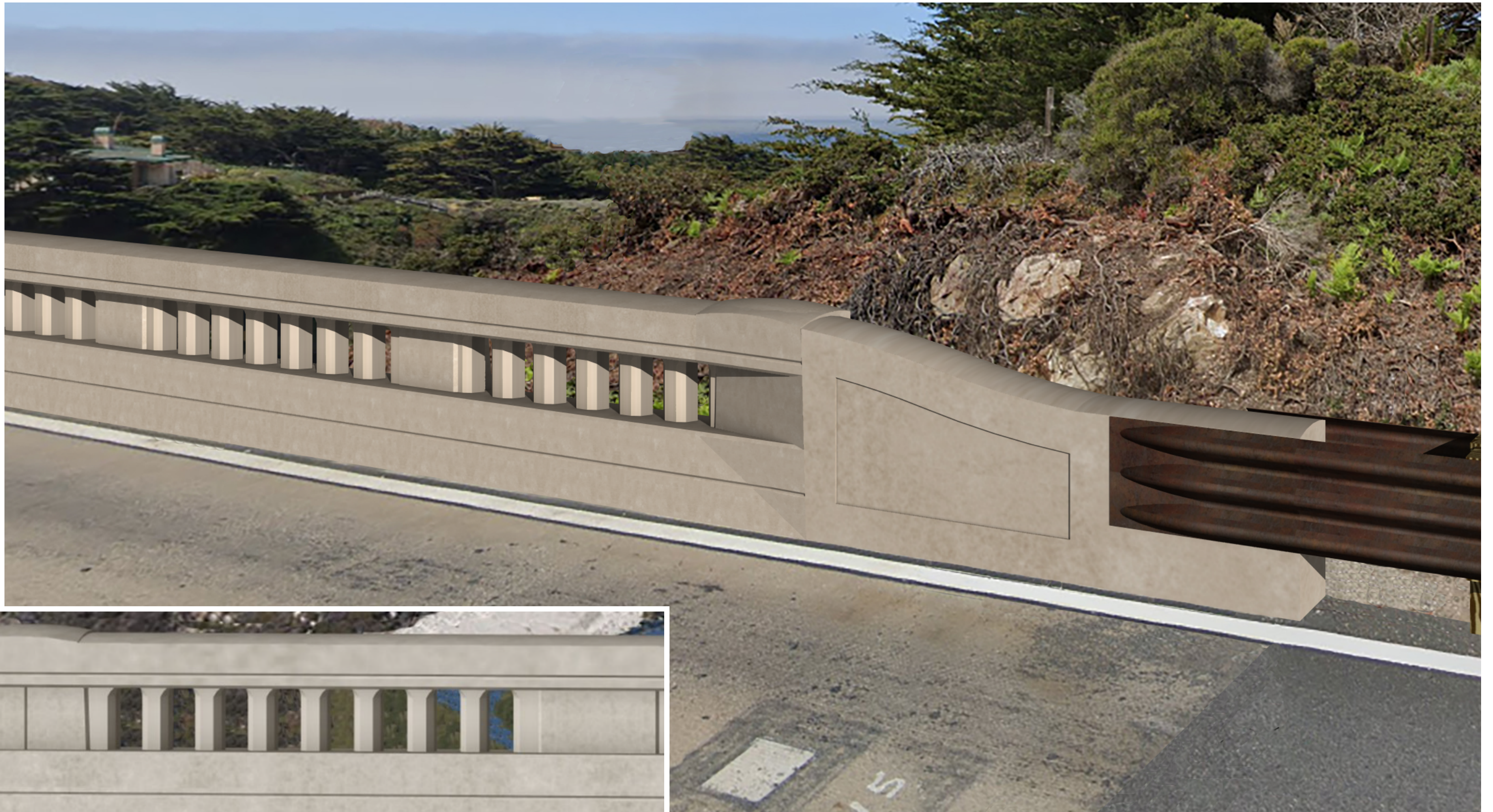
Barrier Alternative - 1 6" Clear Opening with Chamfered Balusters
