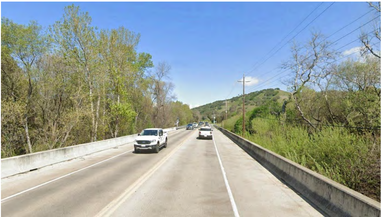
Figure 2.1.10.5 Visual Assessment Unit 4
