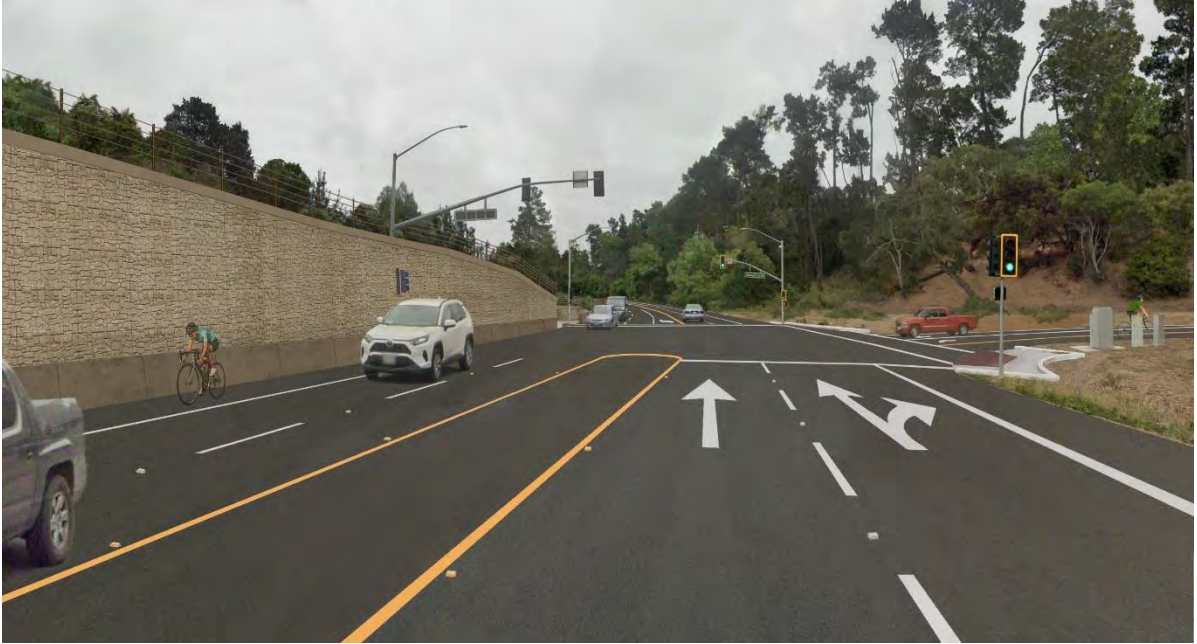
Figure 2.1.10.10 Alternative 2 Signalized Intersection
