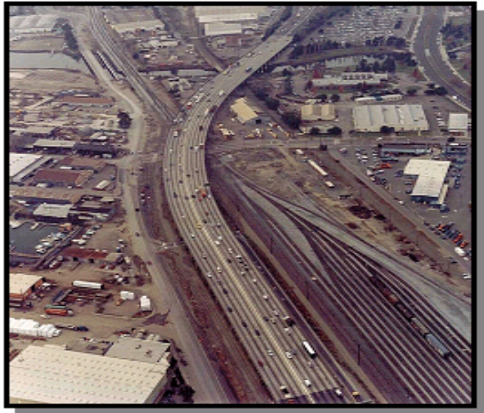
The construction contract is six percent complete.
