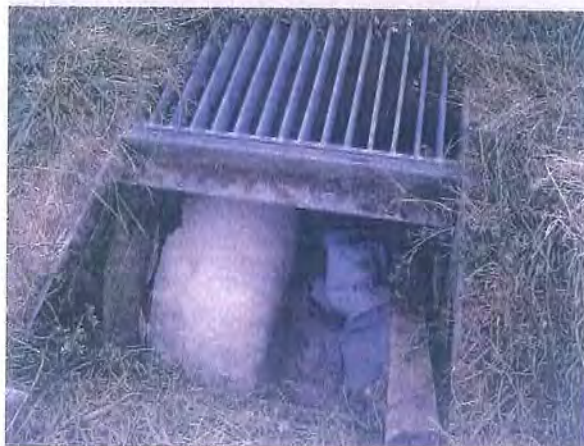
Figure 9 The outlet from culvert C is located in a DI.
