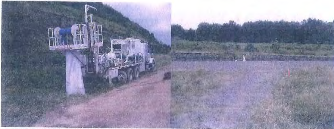
Figure 8 Culvert C is under the eastbound lanes of I-88. The photo on the left show the lining as it enters the culvert. Sample C-1 was taken upstream as indicated. The photo on the right shows the median where the outlet from culvert C is located.
