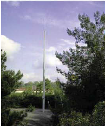
Antenna Installation – Red Bluff
