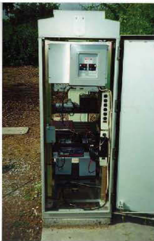
Interior Rear View – Red Bluff
