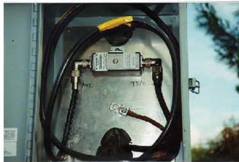
Feedline Lightning Arrester – Red Bluff
