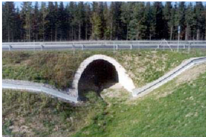
Figure 7. Arch culvert with funneling wall for herptiles and fencing for larger wildlife. Germany.
