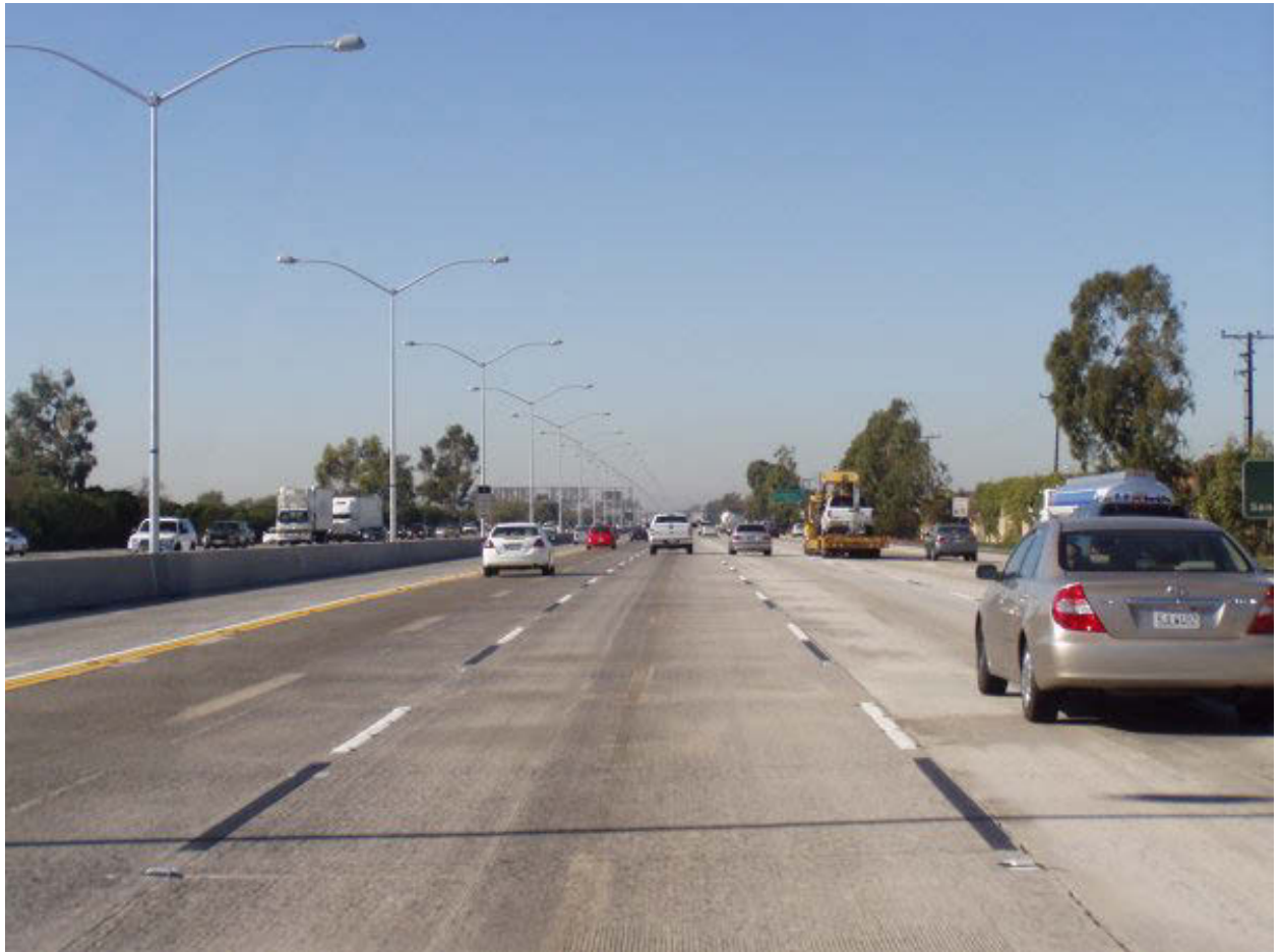
ORA – 405, PM 20.8 / PM 23.1 Median Lighting
