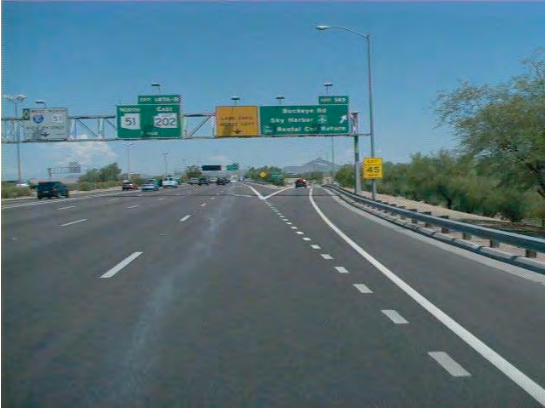
This a sign with the larger route shields and legends as proposed in the new MUTCD.
