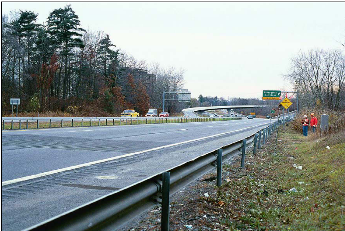
Figure 2. Rumble Strip Reference Measurement Site
