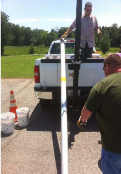
Figure 6. Setting Up Pole for Placement
