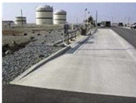
80' Lg x 14' W Concrete Containment Pad Costing over $80,000
