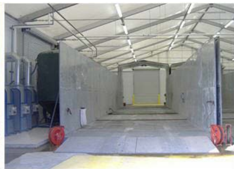
Wash Rack and Treatment System Housed in a Traditional Steel Building
