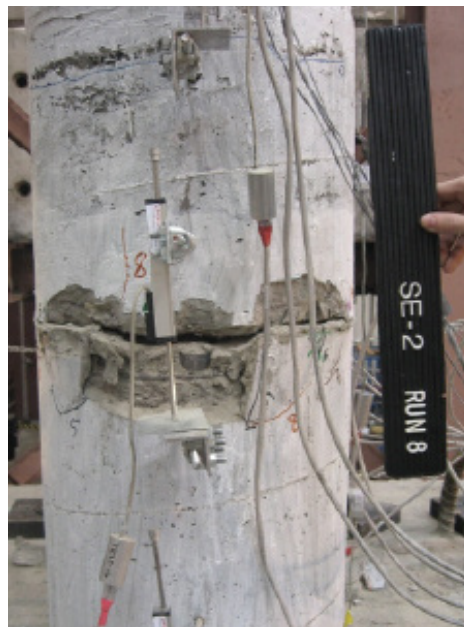
Figure 4: SE-2 (engineered cementitious composite wrapping)
