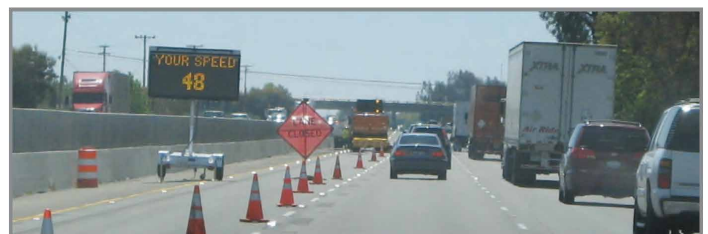
An iCone transmits vehicle speeds to a changeable message sign.
