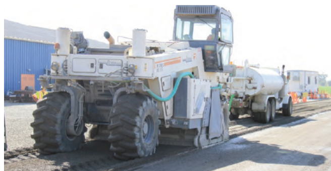
Figure 1: FDR with cement on a test track at UC Davis
