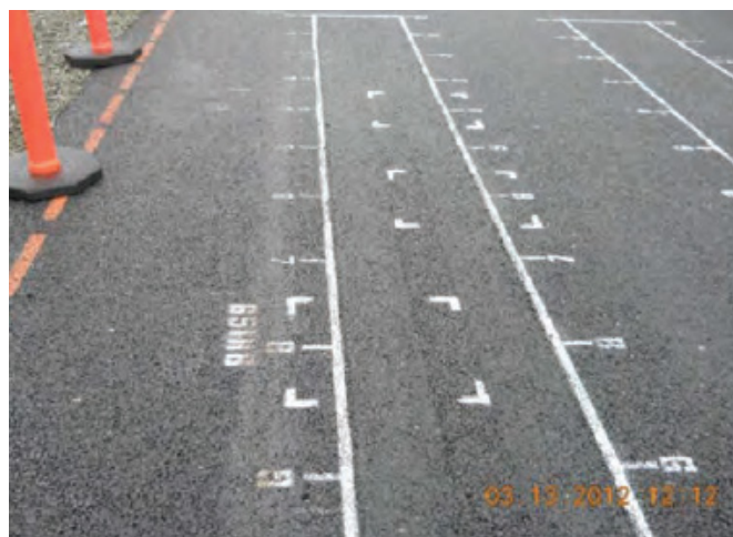
Figure 2: Georgia 1/2-inch mix with PG 58-34PM; OGFC thickness = 0.15 feet
