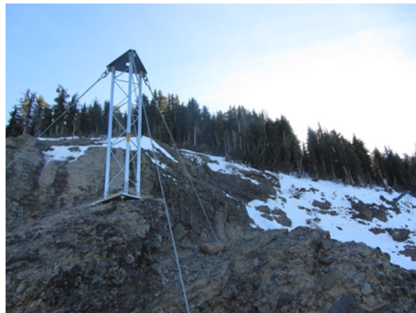
Image 1: Tower installed on Carson Spur to hold the instrumentation equipment
