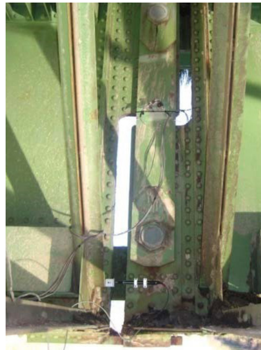
FIGURE 1: Example pin and hanger assembly (Willamette bridge - Oregon)
